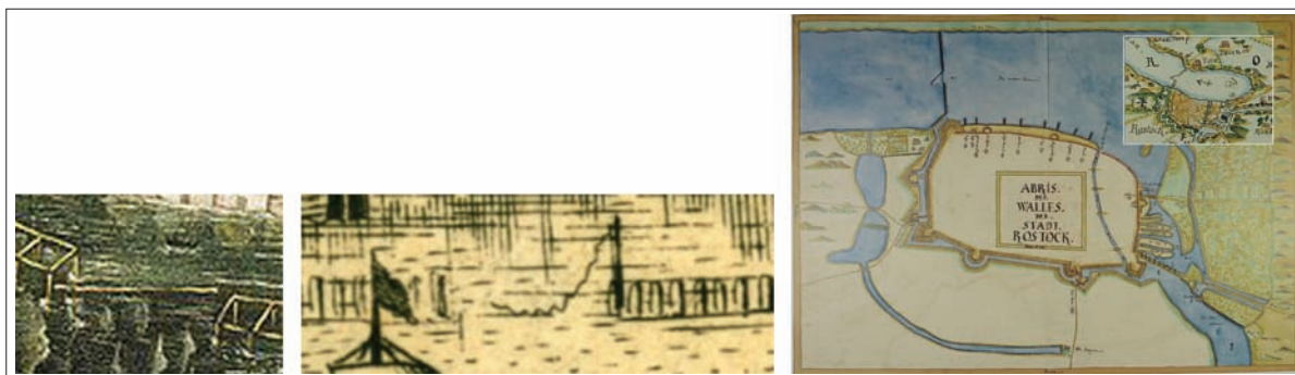
Fig. 15. The gates to the inner harbour were made of two simple constructions: a a simple wooden tree, as seen in this detail of a picture of Stockholm by Olaus Petri, 1535; b, c iron chains were also used, serviced by the 'tree closer' sitting in the tree house, as is visible in a detail from the Merians Wismar illustration from 1653, and the Koinhusens Rostock illustration from the 17th century (Wismar Archive).
